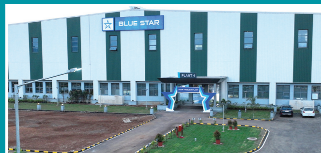
Wada – Deep Freezer Plant
