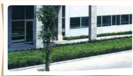
JAPAN Head Office R&D Center and 60 m Height Difference Testing Tower
