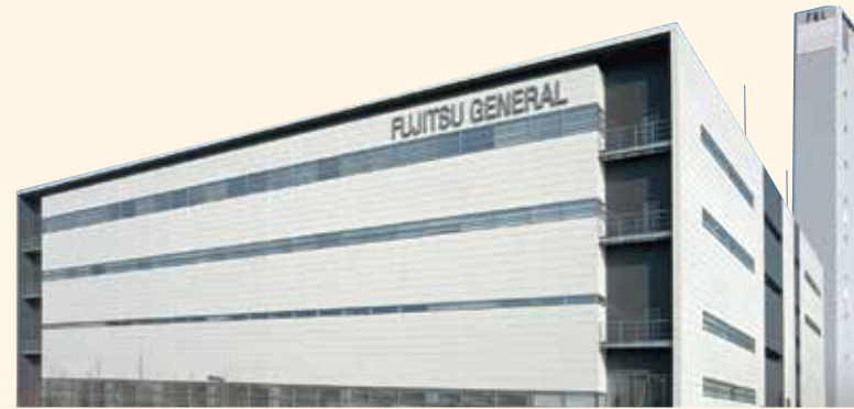
R&D Center and 60m Height Difference Testing Tower
